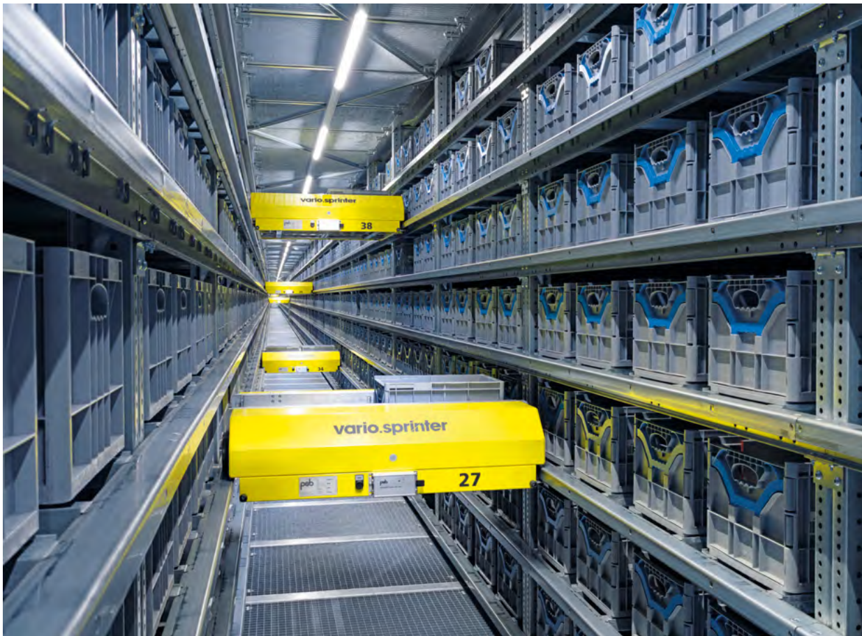
↑ Shuttle warehouse with 150,000 storage locations and a direct conveyor connection at mid-warehouse height
